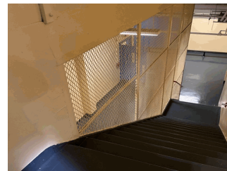
Stair from East Multipurpose Room to Basement
