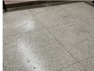
Stair F-G/Basement Exit Vestibule 5
