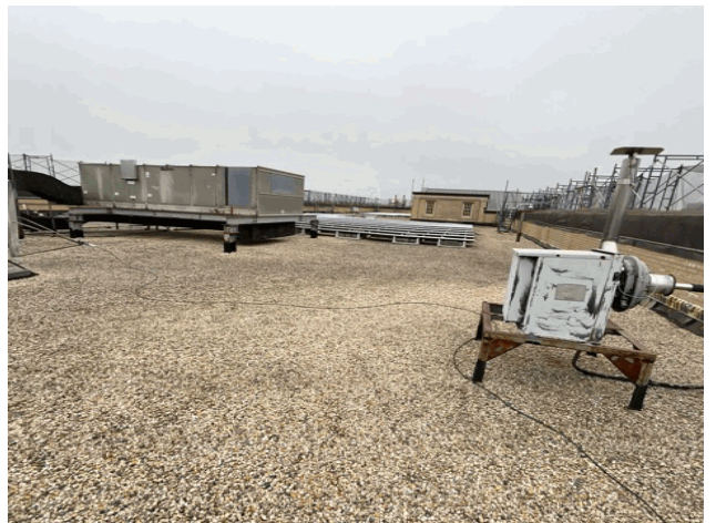
Roof 3 - Southwest View
