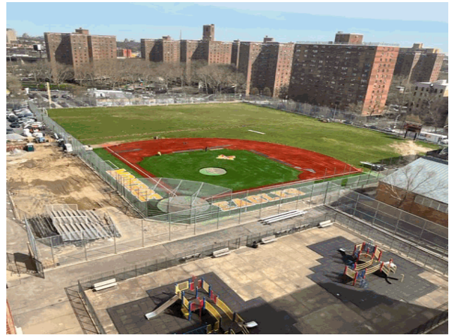
Athletic Field - Northeast View from Main Asset X420
