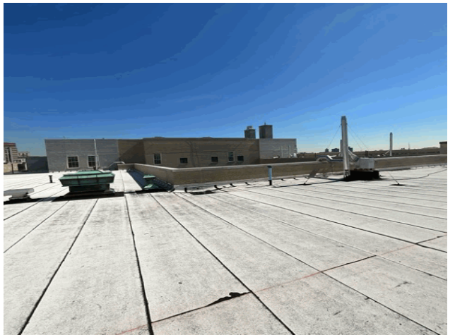
Roof 1 - Northeast View
