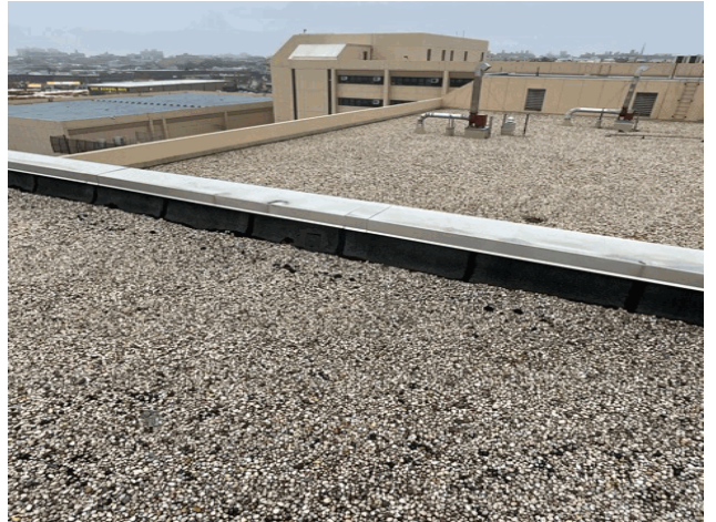
Roof 10 - Southwest View
