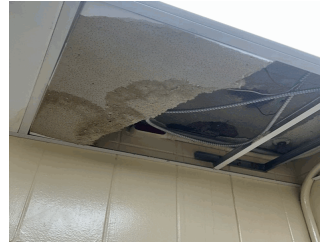
Corridor near Men's Room 176 (Roof 11)
