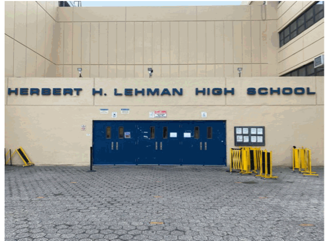
Facade A - East Tremont Avenue
