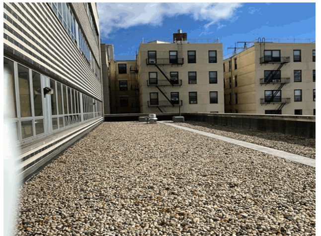
Roof 1 - North View
