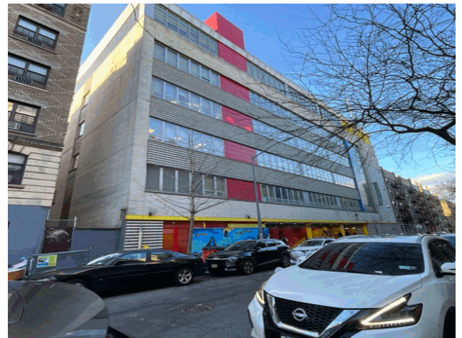
Simpson Street - North View
