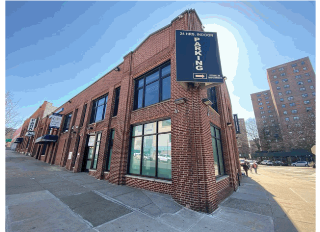
Corner of Broadway and West 230th Street - South View
