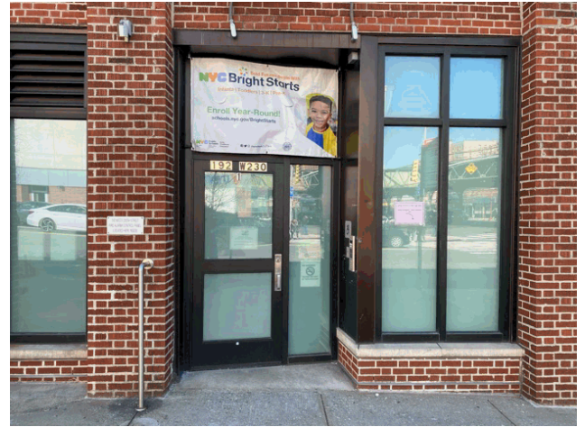
Facade A - West 230th Street
