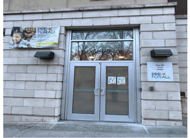
Facade A - Webster Avenue
