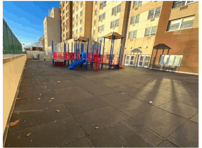
Roof 1 - South View
