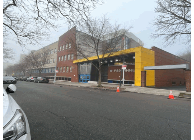
East 211 Street - Southeast View
