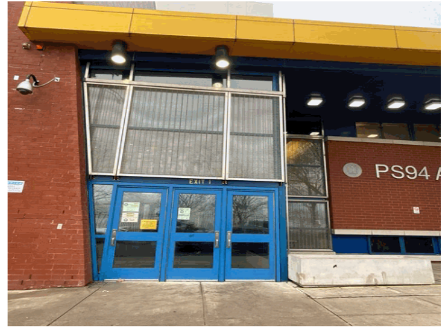
Facade A - East 211 Street
