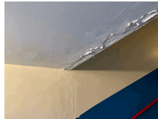
Exit 2 Vestibule shown, also 3rd Floor Elevator Lobby
