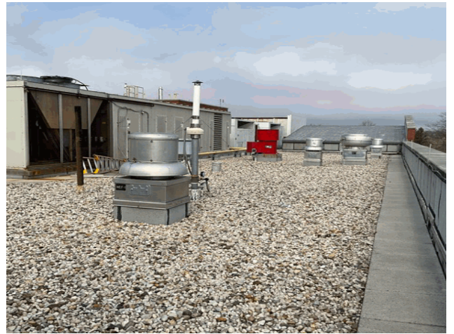
Roof 1 - North View
