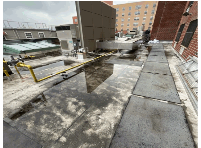
Roof 7 - Northwest View
