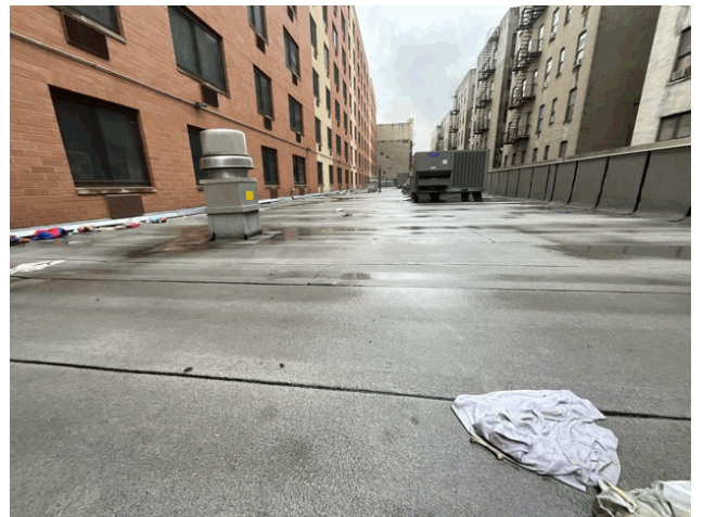
Roof 1 - South View
