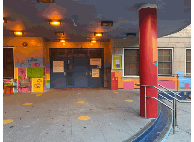
Facade A - West 195th Street
