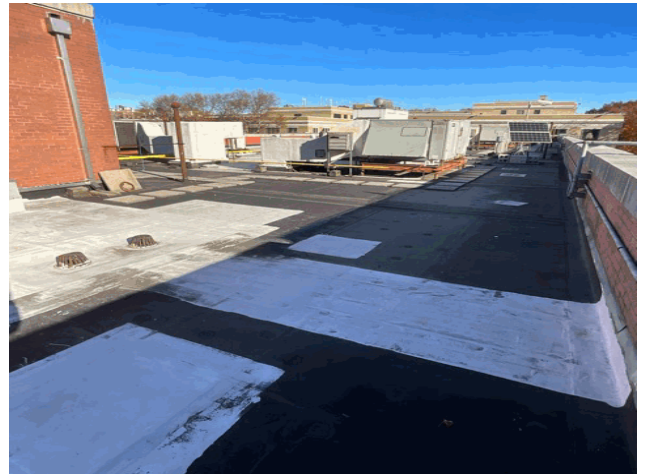
Roof 1 - North view
