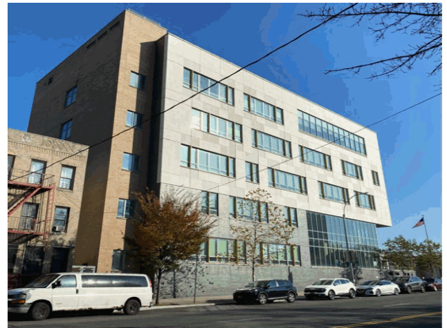
White Plains Road - Southeast View
