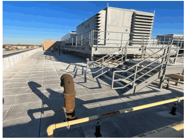
Roof 1 - North View
