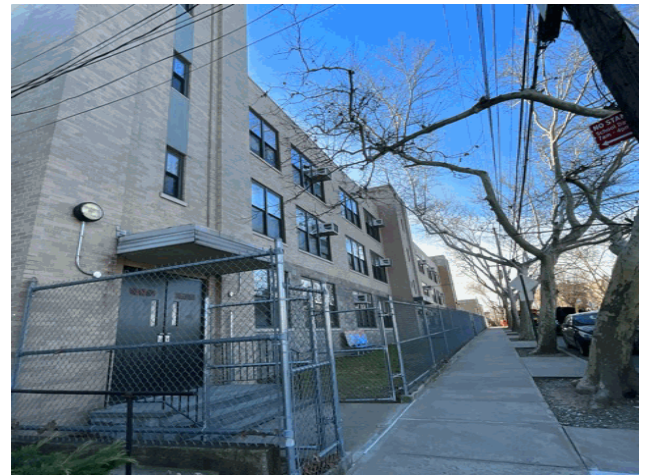
Matilda Avenue - Southeast View
