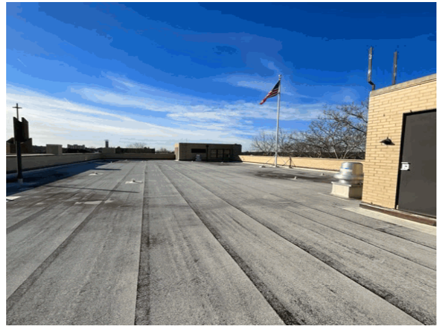
Roof 1 - South View
