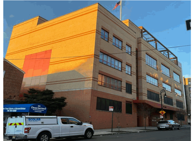
Lydig Avenue - Northeast View
