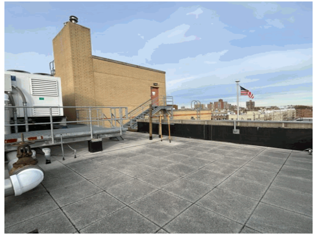
Roof 4 - West View
