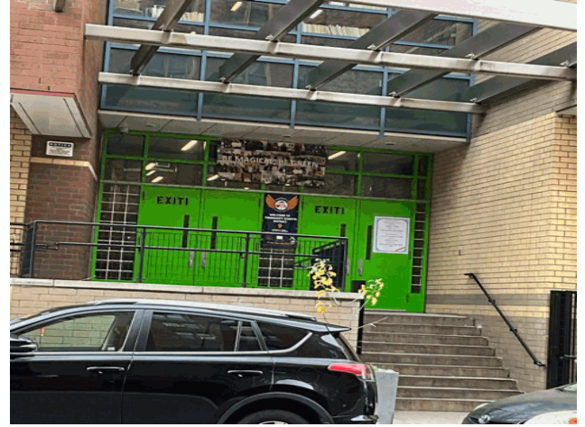
Facade A - West 167th Street
