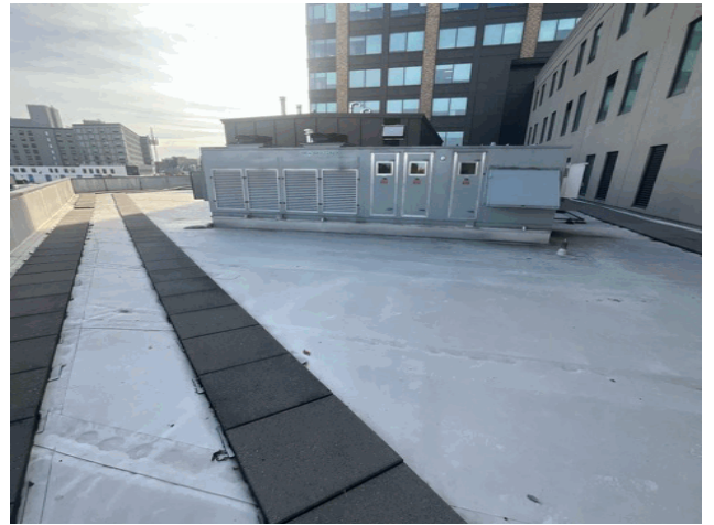
Roof 4 - Southeast View
