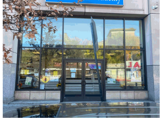
Facade A - Webster Avenue
