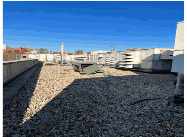
Roof 1 - West View
