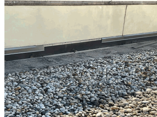
Roof 1 - Facade C
