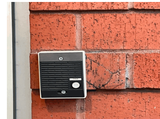
Facade C at Community Entrance Door
