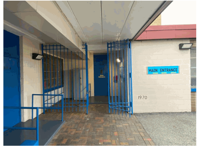
Facade A - East 175th Street
