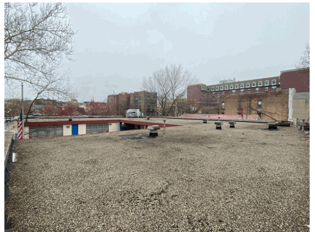
Roof 1 - Northwest View
