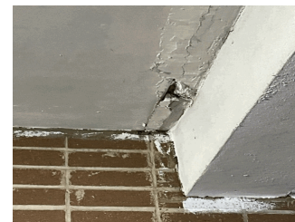
Facade A (above Exit 3)
