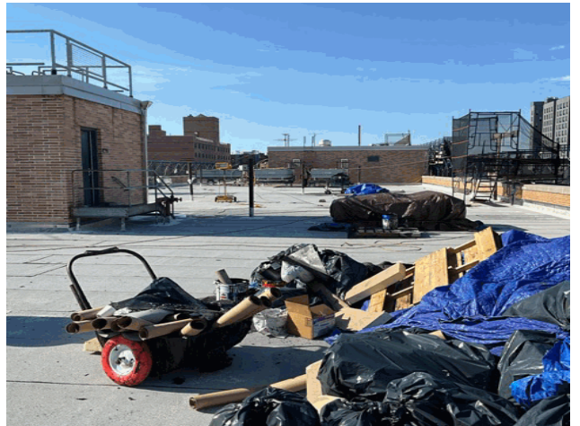
Roof 1 - South View
