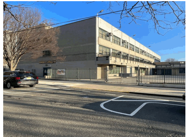
East 179th Street - Northwest View
