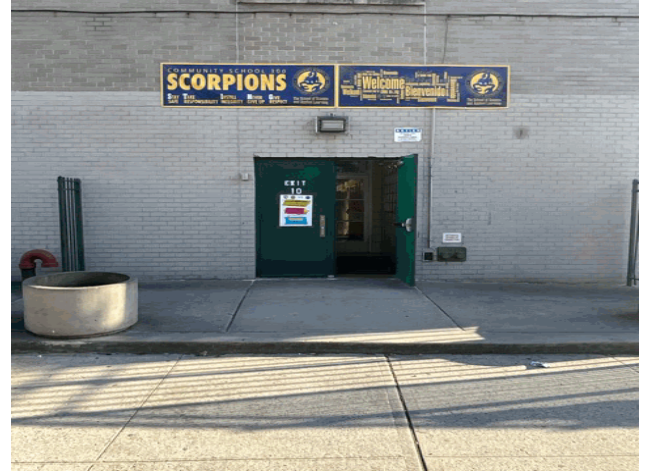
Facade D - Exit 10
