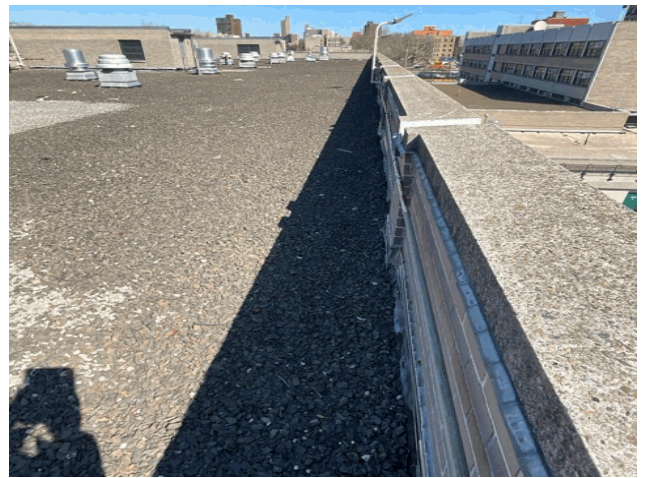
Roof 5 - North View
