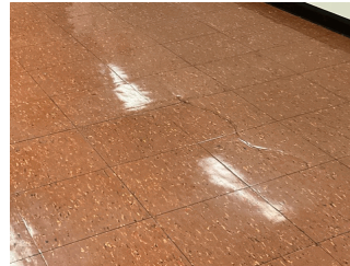
Corridor near Room 414
