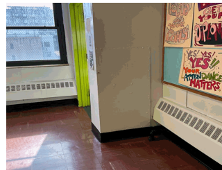
Corridor near Stair B/4
