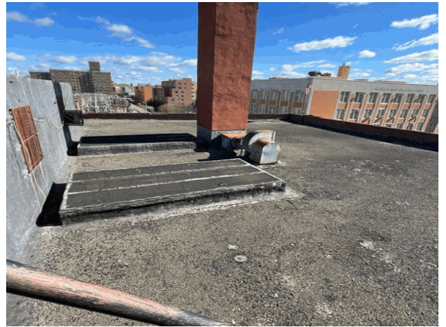
Roof 1 - Northeast View
