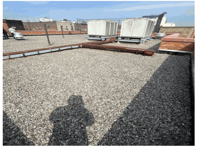
Roof 1 - Northwest View
