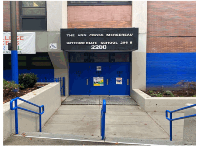
Facade A - Aqueduct Avenue
