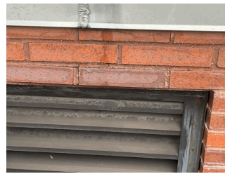
Roof 1 - Chimney CH
