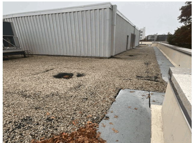
Roof 1 - South View
