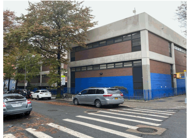
Corner of Aquaduct Ave and West 183rd Street - Northeast View
