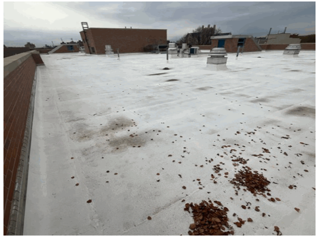
Roof 1 - Southwest view
