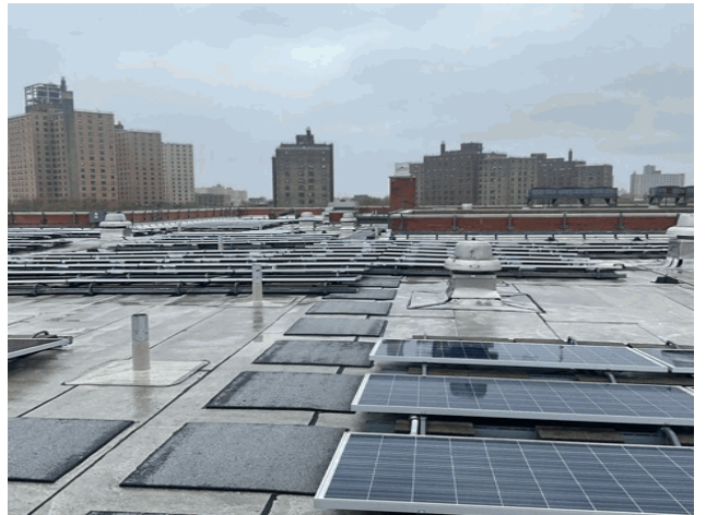
Roof 1 - South View
