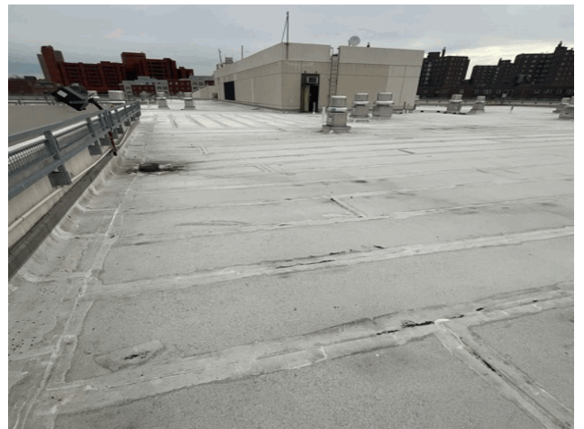
Roof 1 - North View
