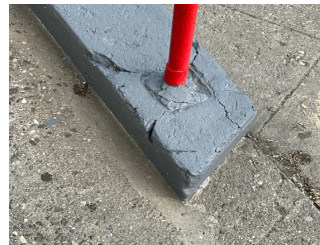
Service Ramp to (Exit 9)
