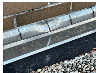
Roof 1 - Facade B
