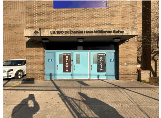
Facade A - North View
