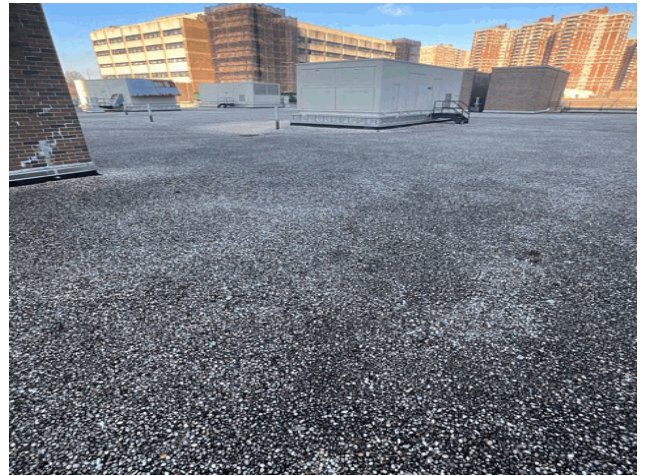
Roof 1 - Northwest View
