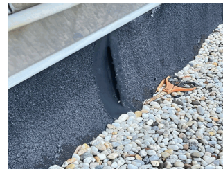
Roof 1 - Facade D
