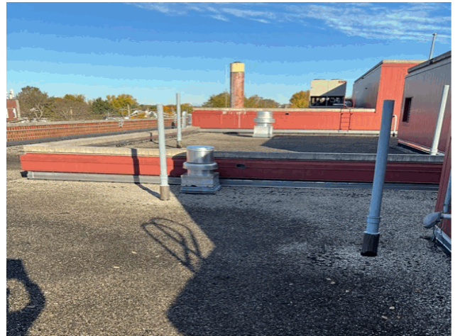
Roof 1 - South View
