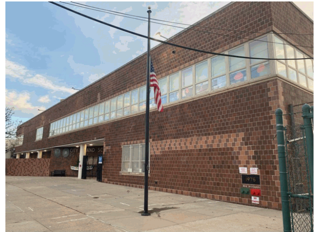
City Island Avenue - Northeast View
