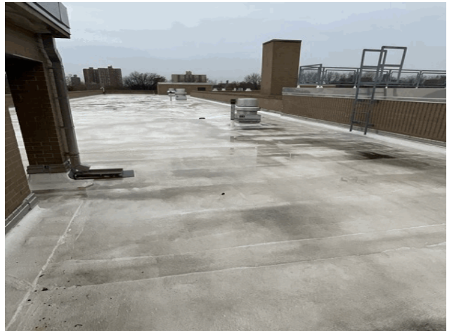
Roof 1 - North View
