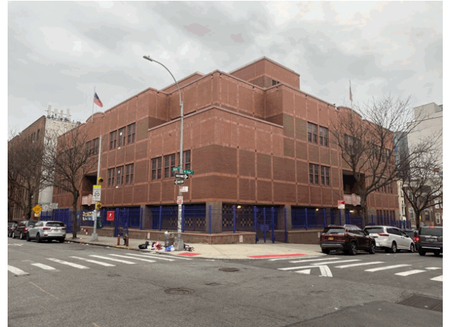
Corner of Walton Avenue and Mt. Hope Place - Southwest View
