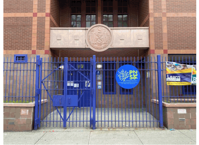
Facade A - Walton Avenue
