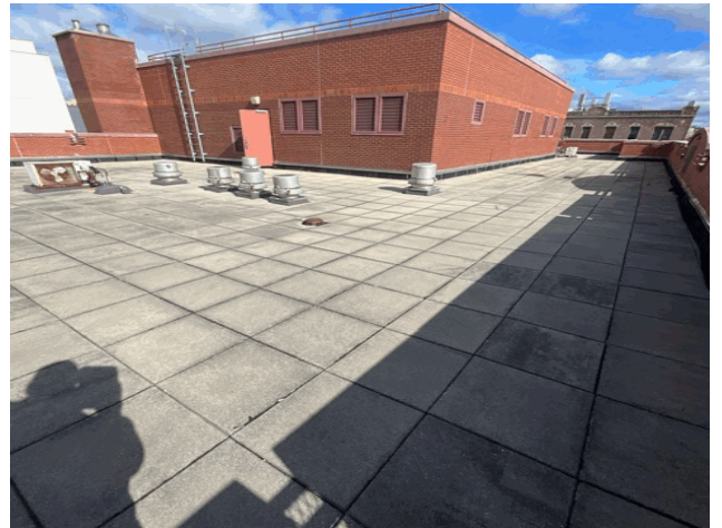
Roof 1 - Northwest View
