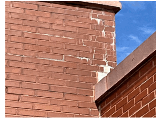
Roof 1 - Chimney CH
