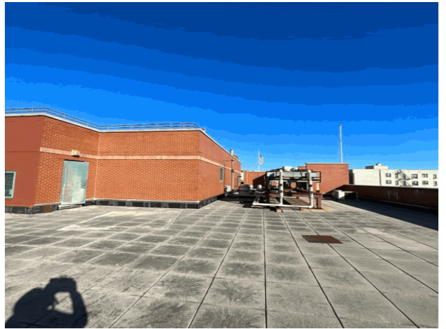
Roof 1 - Northeast View
