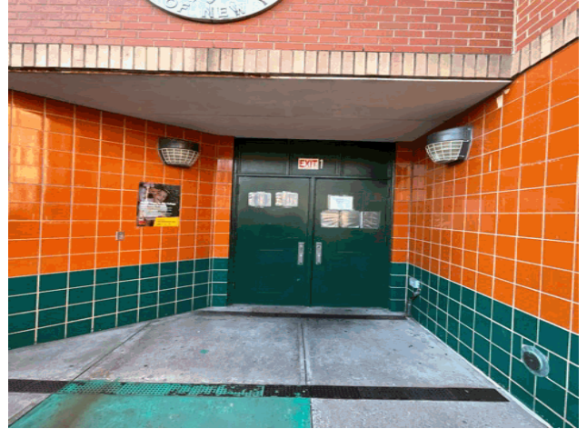
Facade A - West 171st Street
