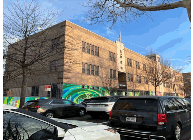
Fulton Avenue - Southeast View
