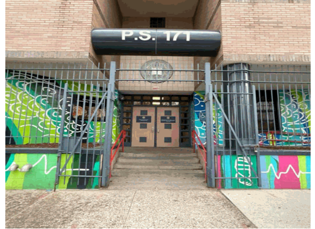
Facade A - Fulton Avenue
