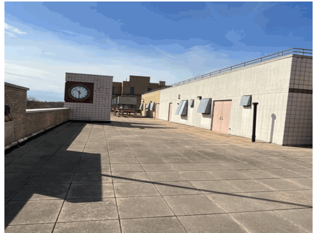
Roof 1 - South View
