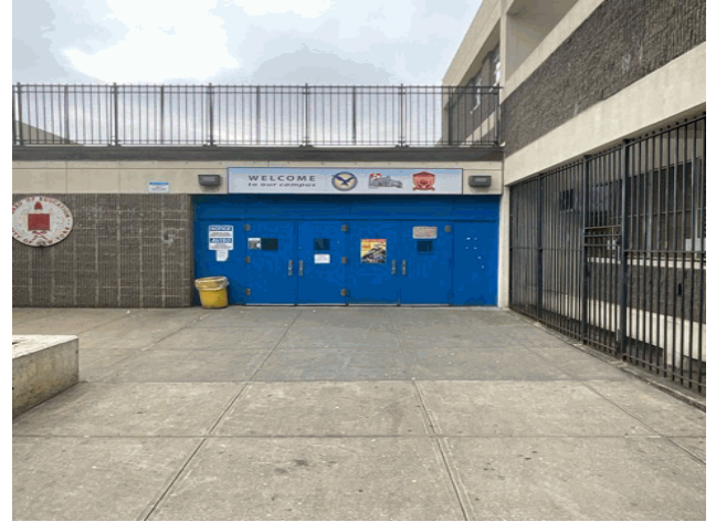
Facade A - West Farms Avenue
