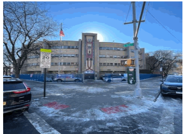
Corner of East 164th Street and Grant Avenue - South View
