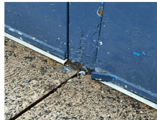
Facade C at Exit 6
