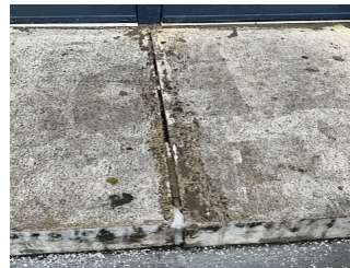
Facade D at Exit 7
