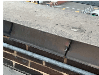
Roof 1 - Facade A
