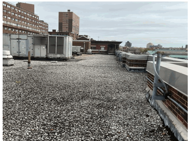
Roof 1 - West View
