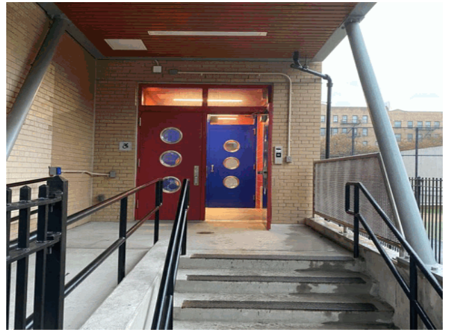
Facade A - Tinton Avenue
