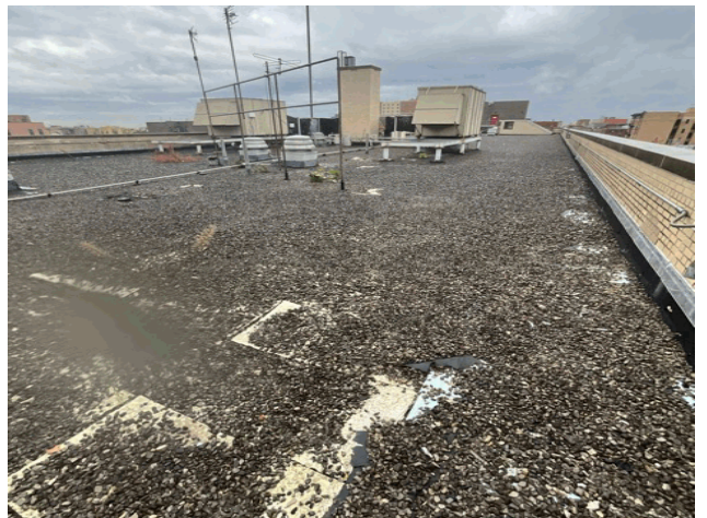
Roof 1 - South View
