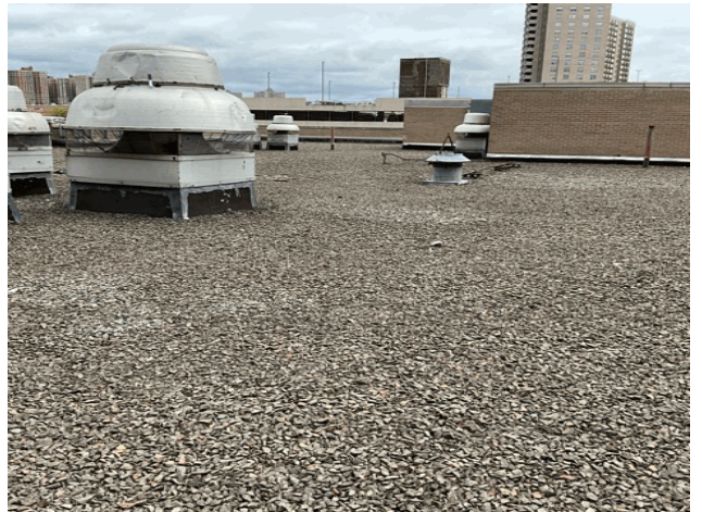
Roof 7 - Northwest view
