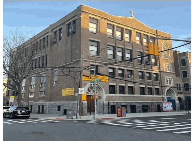
Corner of Washington Avenue and East 183rd Street - Northwest view
