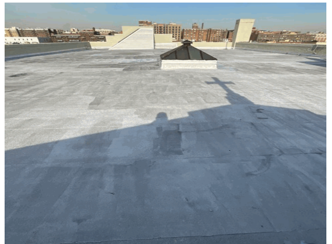
Roof 1 - West View
