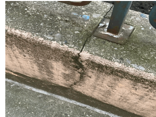
Facade A - HC Ramp
