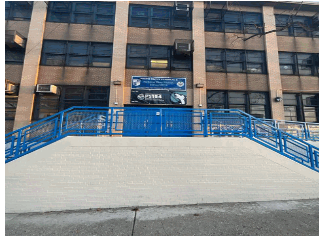
Facade A - East 135th Street
