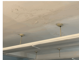
Room 302C, also Room 302D and Corridor near Room 302C
