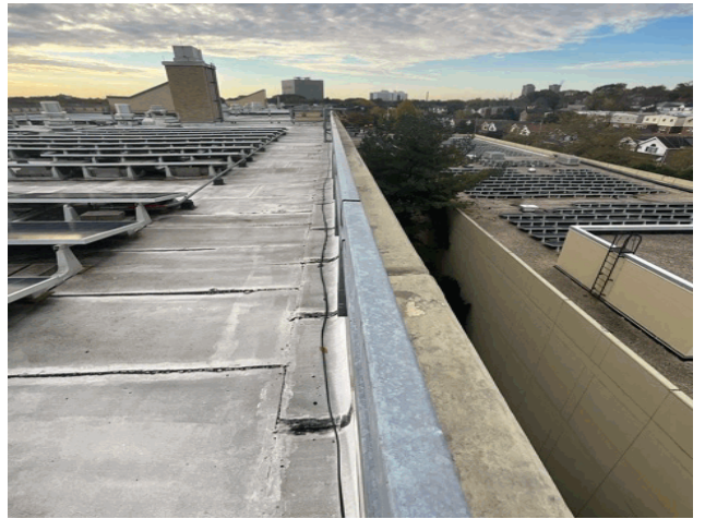
Roof 1 - South View
