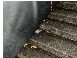
Stair near Exit 6
