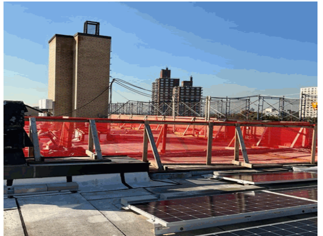
Roof 1 - South View
