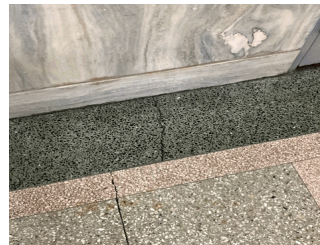
Main Entrance Lobby
