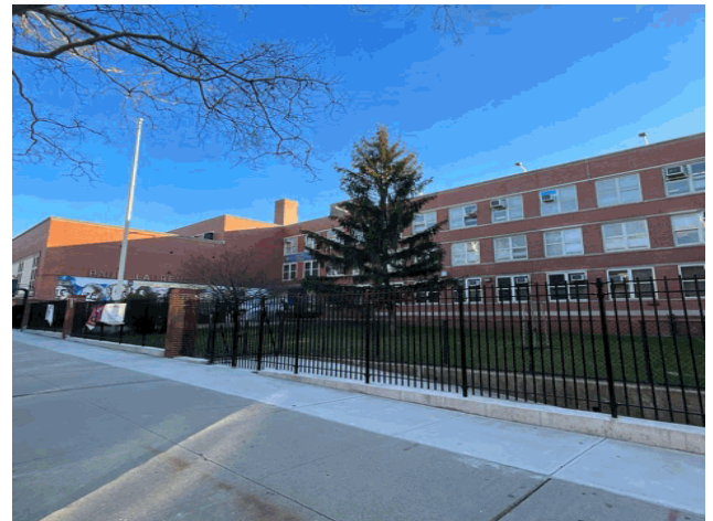
Cauldwell Avenue - Northeast View
