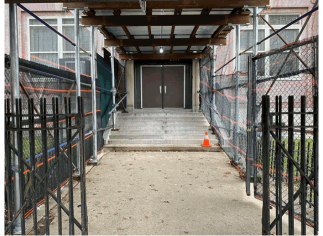
Facade A - Pugsley Avenue
