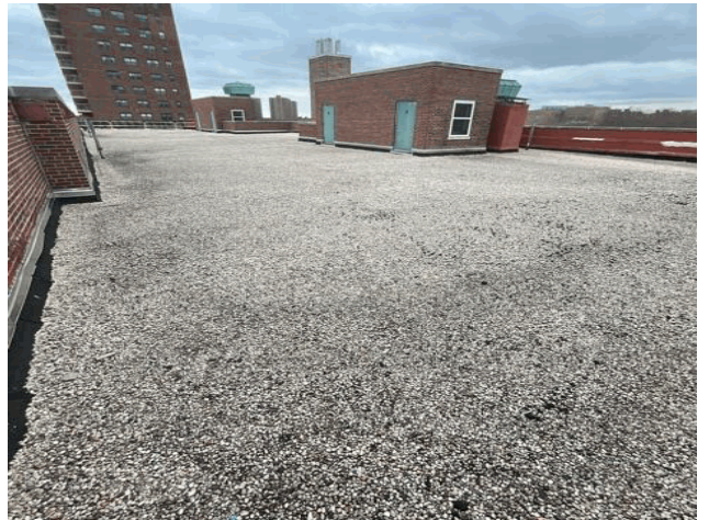
Roof 1 - Southwest View
