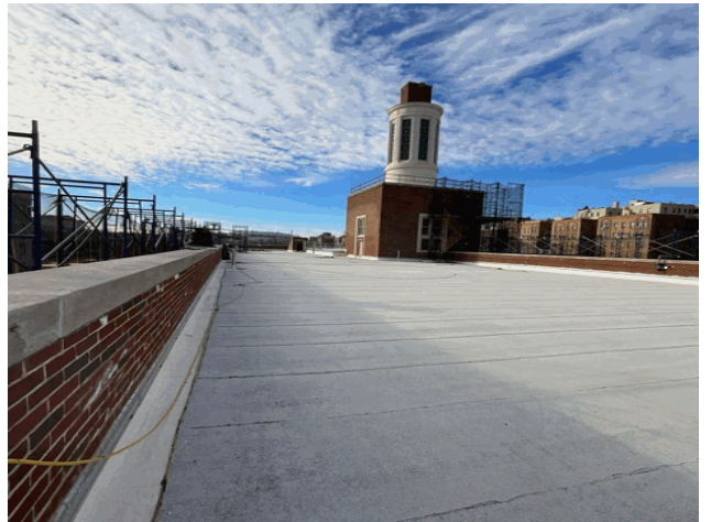
Roof 2 - North View
