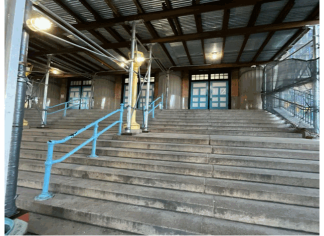
Facade A - Barnes Avenue
