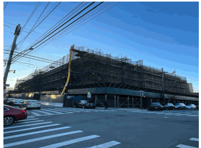
Corner of Barnes Avenue and East 217th Street - Northeast View
