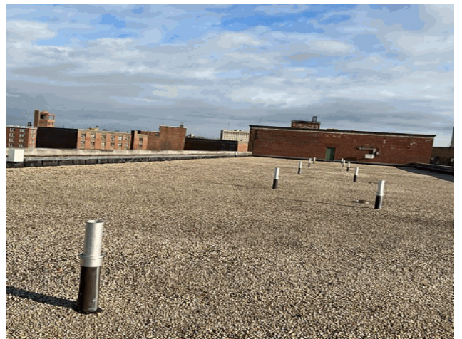
Roof 3 - Northeast View
