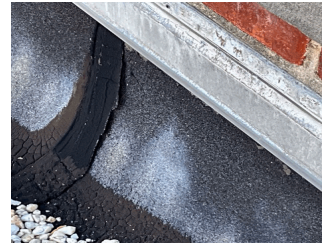
Roof 3 - Facade A
