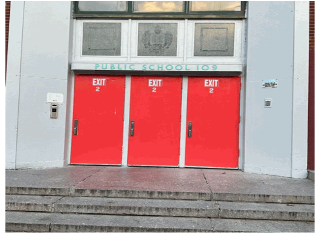
Facade A - Popham Avenue
