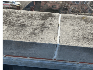
Roof 3 - Facade A
