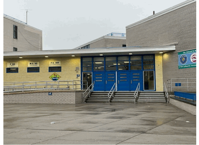
Facade A - Lafayette Avenue
