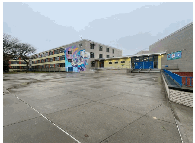
Lafayette Avenue - Northeast View
