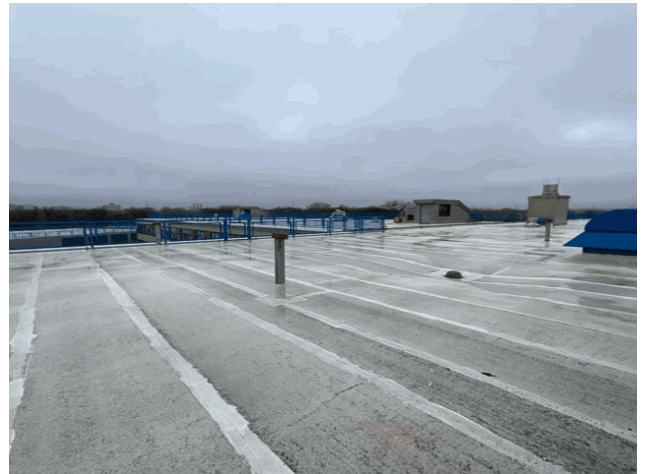
Roof 1 - Southwest View
