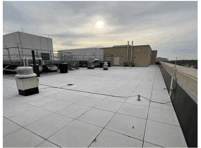
Roof 1 - South View
